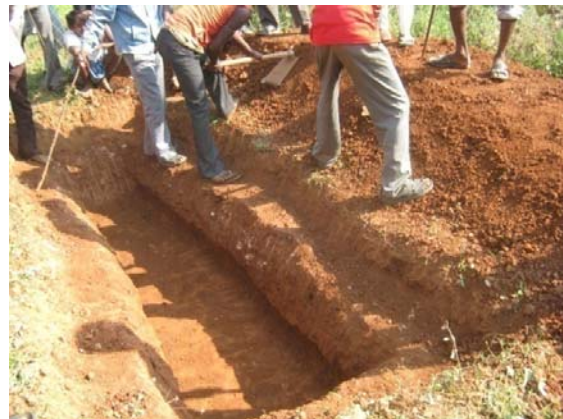
Construction of Rain Water Harvesting Structure in the Field
